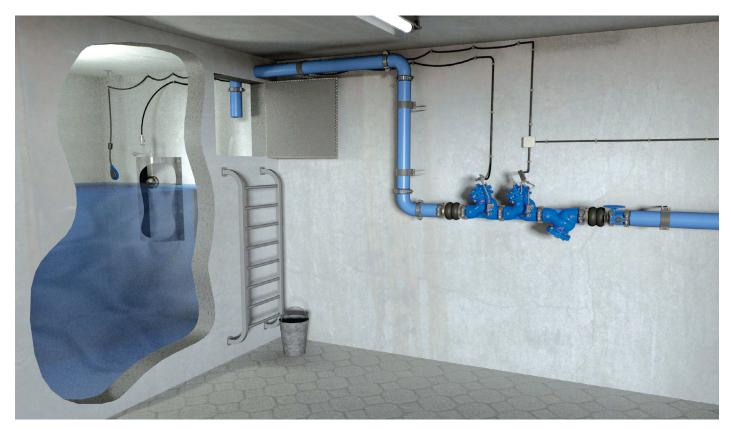
**Water Reservoir Level Control System**, featuring the BC-750-67-P that maintains constant water level in the reservoir. As backup another level control valve is stationed upstream and calibrated to a slightly
