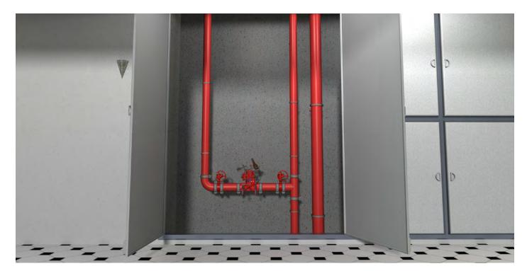
BERMAD BC-791-F0 featured as floor breach containment valve - it will remain fully open under no flow conditions or when supply of fire water to downstream wet pipe system is needed, should downstream pipe line fail, the excessive flow will automatically close the BC-791-F0
