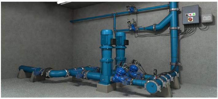
The BERMAD BC-730-P As a pressure sustaining valve that recycles water back to the reservoir at stagnate pump operation, it will remain close when raiser pressure is normal. In an event where the pump works at low flows and high head, the BC-730-P will open to allow sufficient water circulation and pump cooling.
