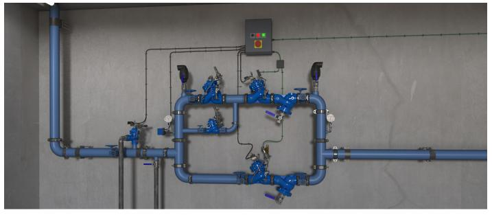
**Pressure Reducing Station** with Block Valve and Automatic Backup. In case of abnormal pressure rise detected by the PS the system switches
