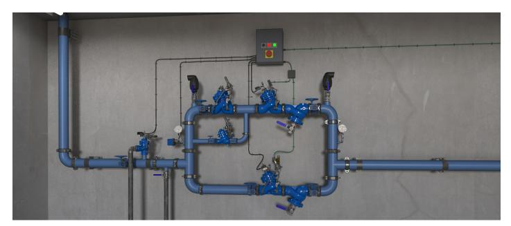
**Pressure Reducing Station** with Block Valve and Automatic Backup. In case of abnormal pressure rise detected by the PS the system switches
