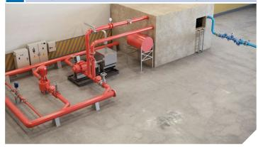
Basement pump room - Reservoir level control with overflow protection, fire protection pumps system with pressure relief valves optional for direct pumping - Suction Control.
