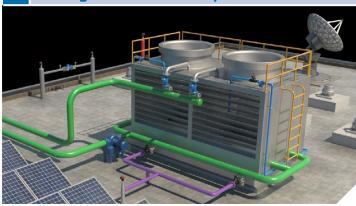
Cooling towers system - Control Valves for Make-Up water, Balancing and Controlled Bleeding.
