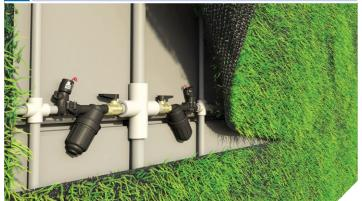
Vertical Irrigation Valves array - utilizing condensate from the cooling towers the system provides regulated pressure and complete control of irrigation in multiple pressure zones.
