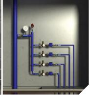
On Floor system supply, Reducing valve for Potable water.
