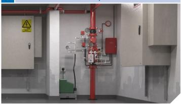
Fire Protection System for elevator machine room, Pre-Action System, Protection with minimal water damage risk.
