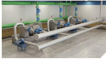
Chillers machine room, individual Chiller Flow & shut off Control, Energy measurement. Balancing between Supply and Return by pressure differential control at end of circulating lines (roof top). Cooling Towers return line flow balance.
